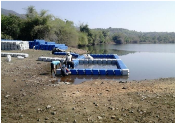
Assembling and Installation of cages in the Chapoli Reservoir
